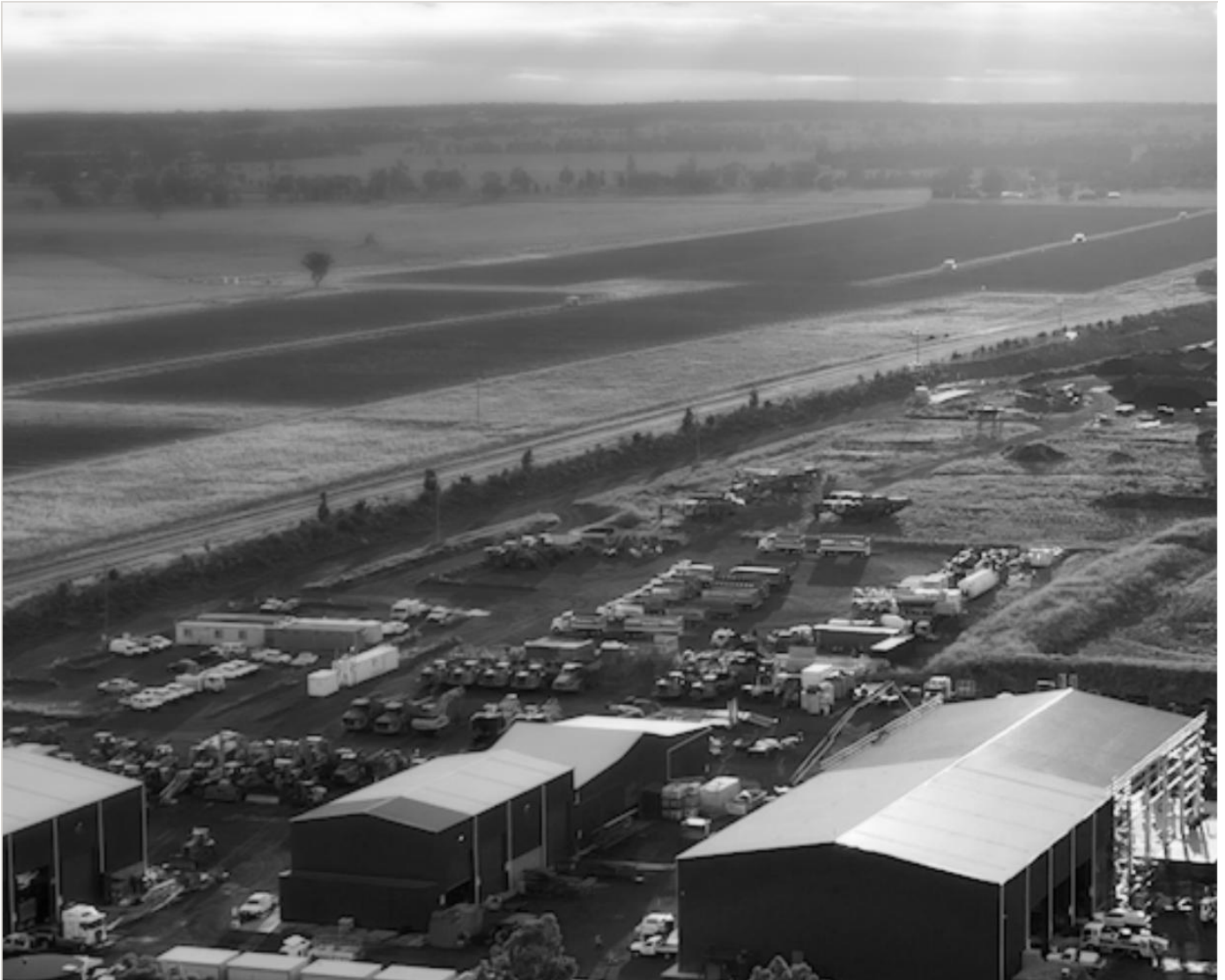
Construction Materials operations. Official FY2025 annual-report image. Source
